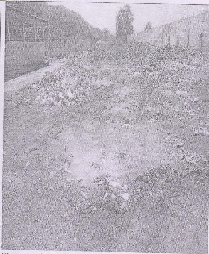
Photograph No. 8 –Shows Status ofleachate generated from Solid Waste
